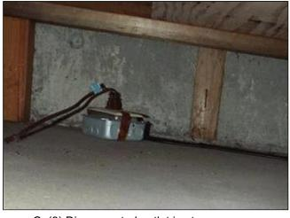
C. (3) Disconnected outlet in storage room.
