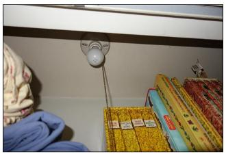
D. (3) Open bulb fixture in hallway closet.
