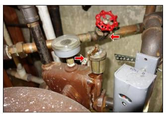
A. (3) Water leaks at main water shut-off valve and air bleeder valve on boiler.
