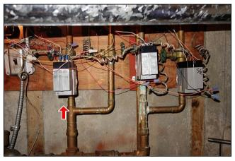
B. (1) Malfunctioning switch to bedroom zone heating.
