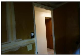
E. (1) Garage door does not have self-closing mechanism.
