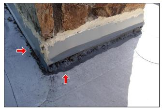
B. (1) Foam filler on chimney flashing.
