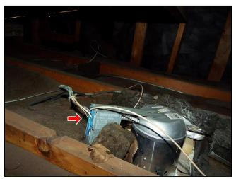
D. (4) Missing bushing where wires enter can light housing in attic.
