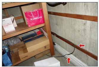
C. (2) Outlet and wire disconnected from wall in storage room.
