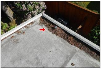
D. (1) Debris collecting around gutter downspouts on roof.
