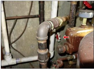
A. (1) Main water shut-off behind boiler.
