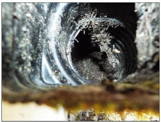
D. (3) Gutter drain pipe full of debris.
