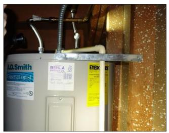
D. (1) No thermal expansion tank on hot water heater.
