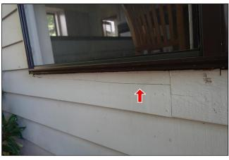
A. (2) Siding cracks below kitchen window.
