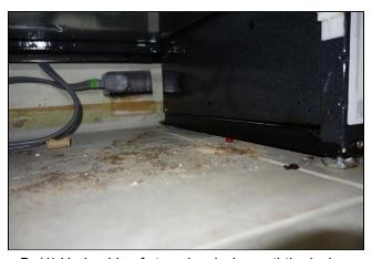
B. (1) Underside of stove is missing anti-tip device.
